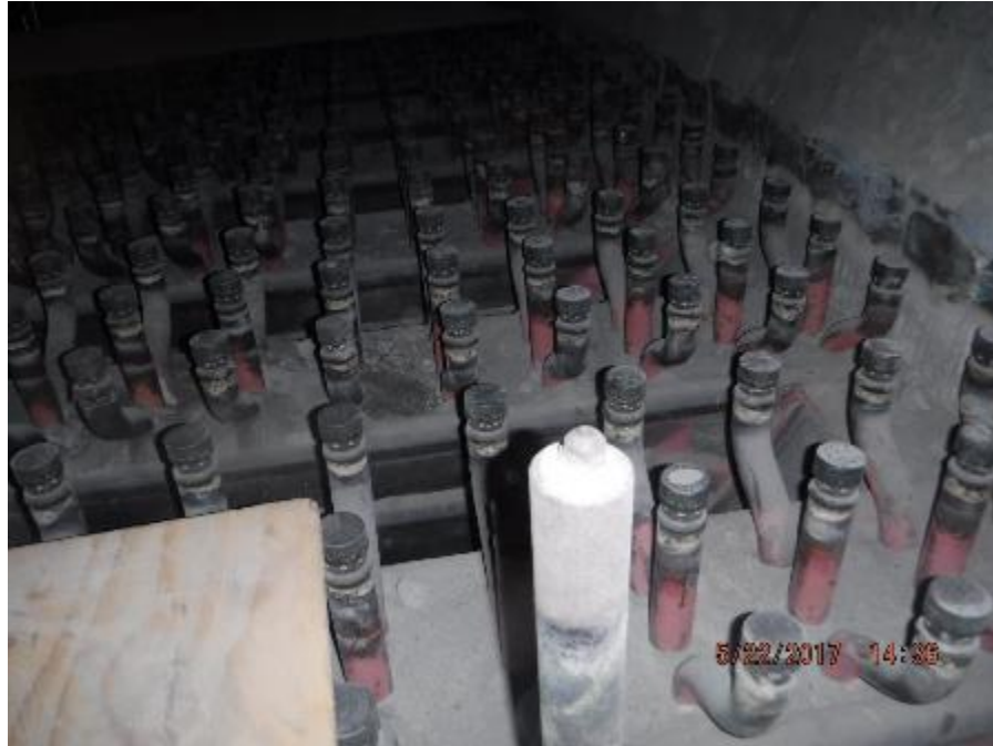
Photo 62 – Lower furnace single TC are in good condition.
