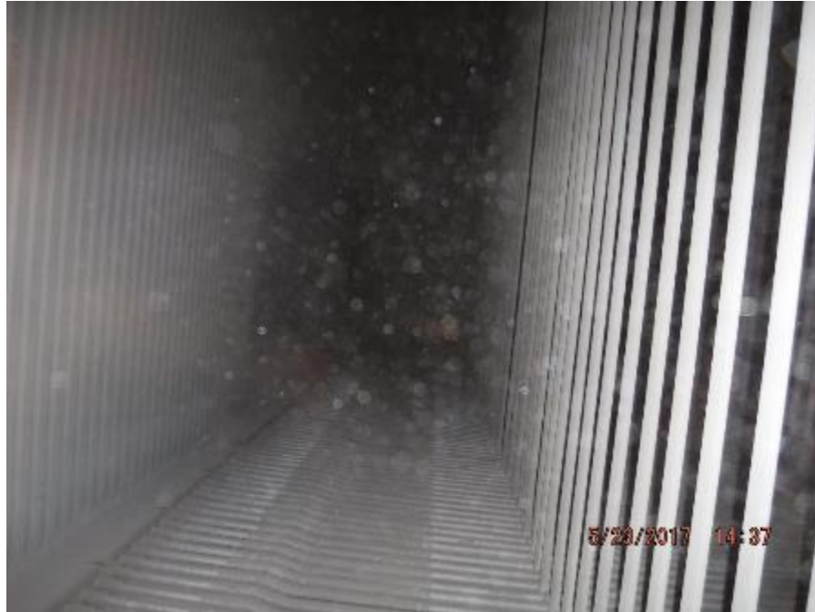
Photo 32 – Rear row of SH stringer tubes are straight and in plane.
