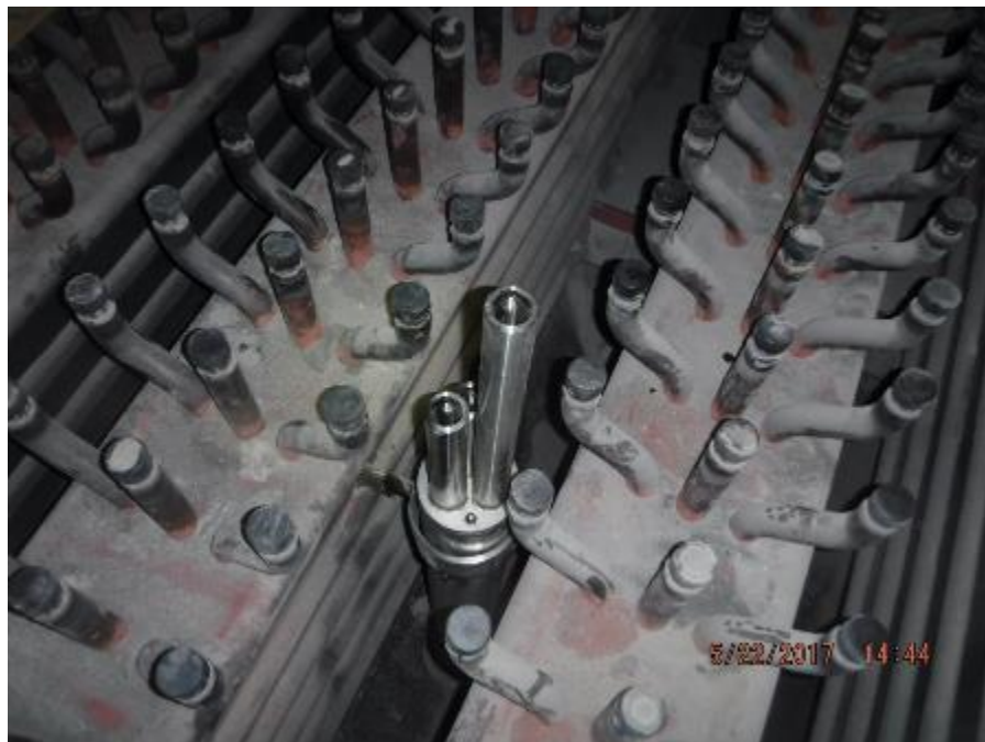
Photo 63 – Lower furnace, three staged TC replaced.
