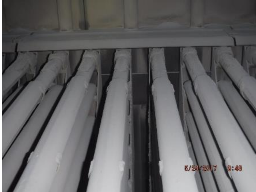
Photo 6 – Front wall supports for boiler bank elements are in good condition.
