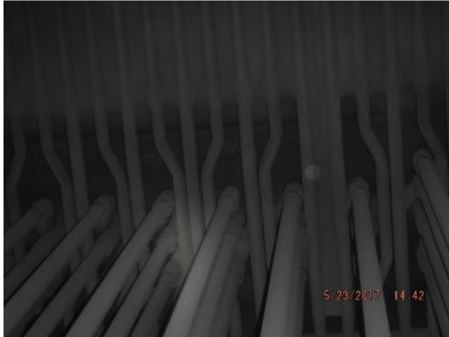
Photo 23 – View of roof tubes above rear wall screen tubes.
