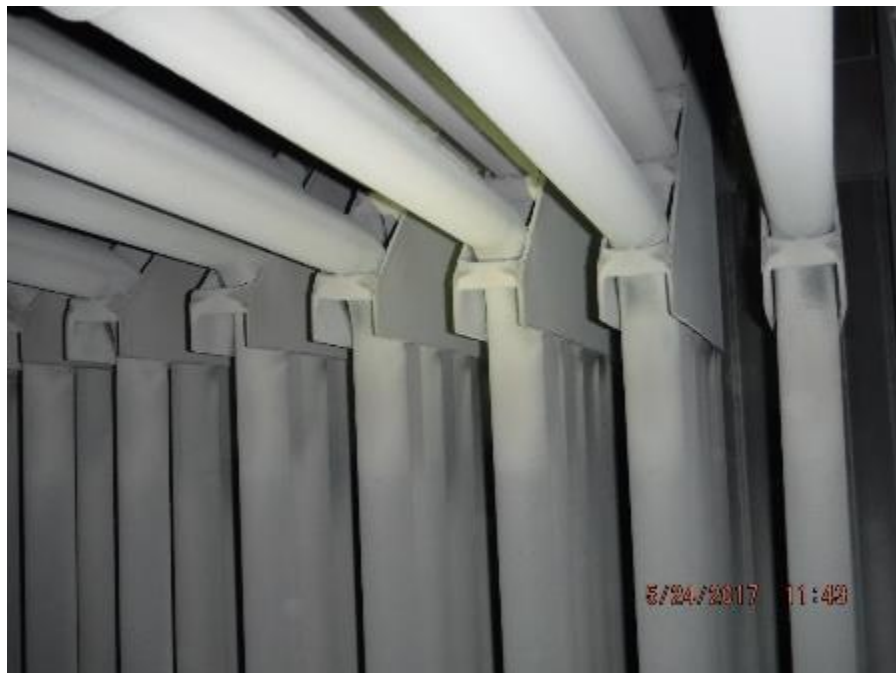
Photo 7 – Rear wall supports for boiler bank elements are in good condition.
