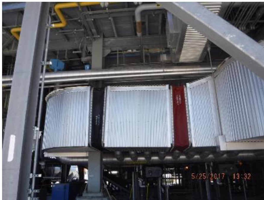
Photo 71 – Expansion joints replaced on PA supply duct.
