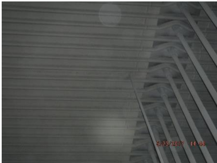
Photo 24 – View of back pass roof tubes.
