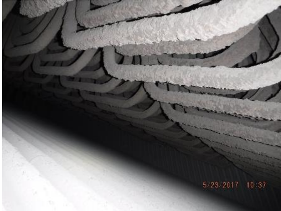
Photo 55 – Finishing SH; view of lower tube loops.
